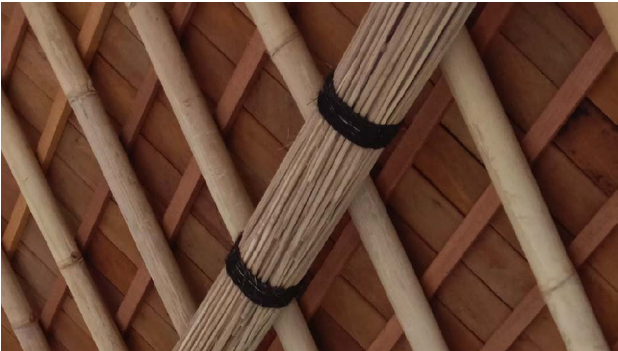
Bamboo lidi beam supporting the rafters and the roof. RASLI villa, Ubud, 2020.
