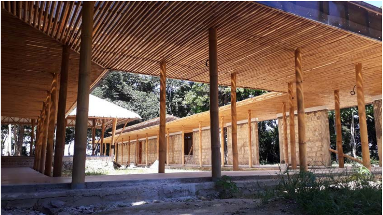
Bamboo tali poles Ø 6-7cm for cladding – Boyoma, Republic of Congo. 2016.
