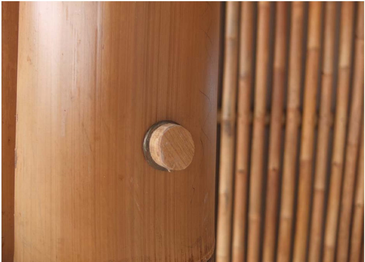
Cover of the steel bars with bamboo caps – Yoga Shala, Joali Being, Bodufushi, Maldives, 2021.
