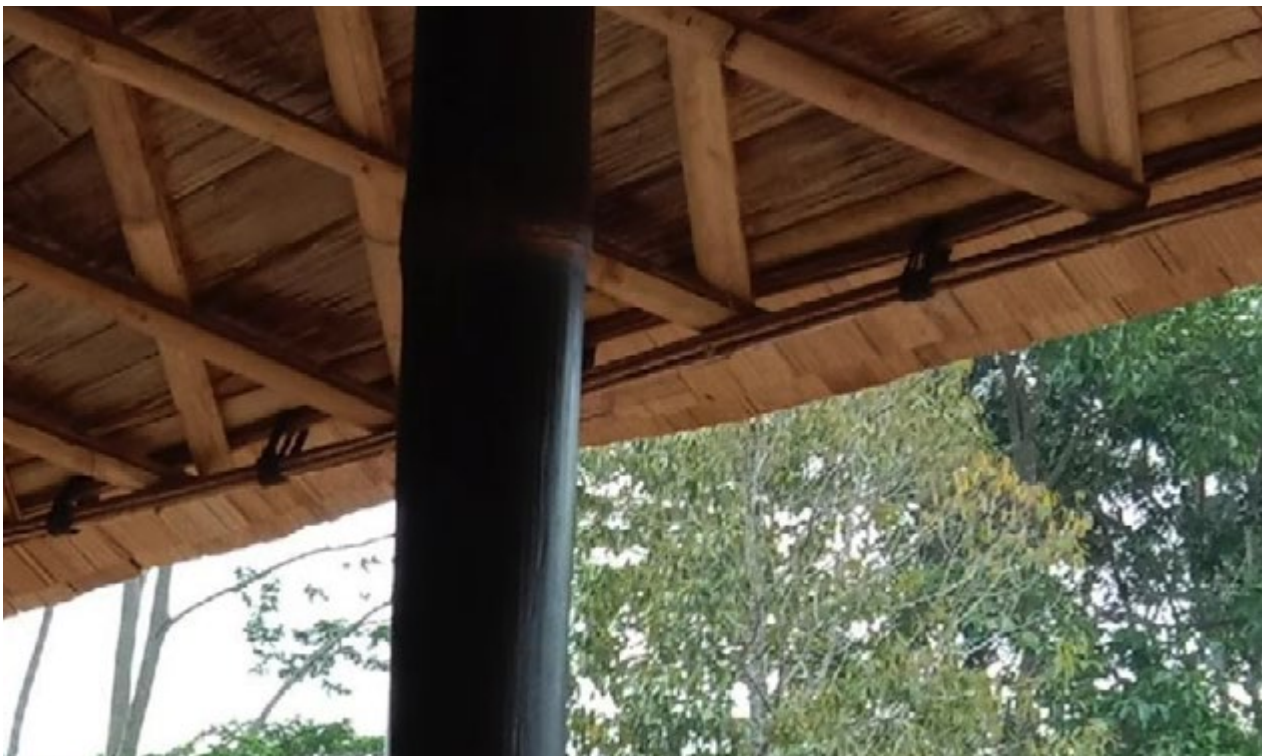
Bamboo lidi roof edge – K Club lobby – Tegallalang, Bali. 2019.
