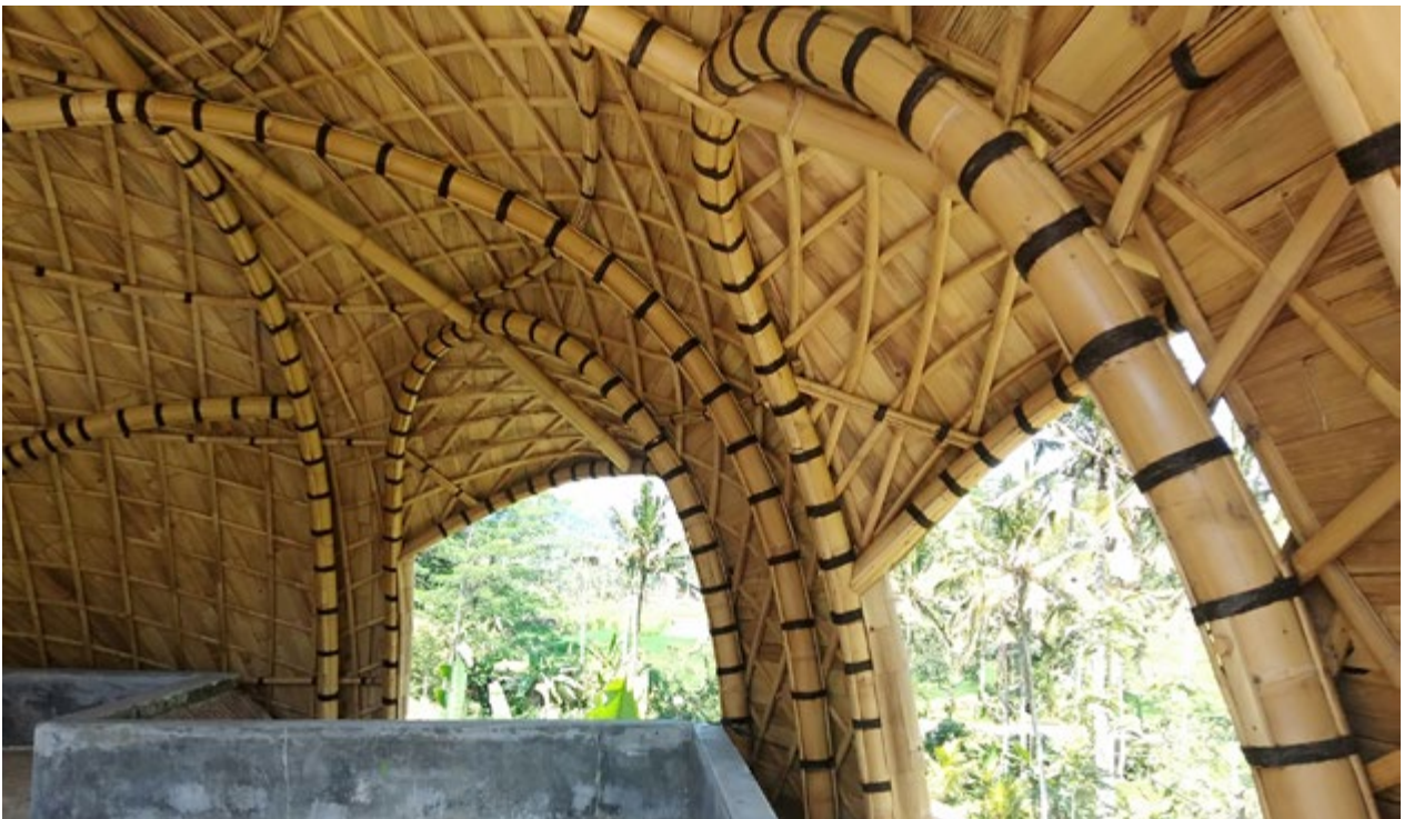
Round Bamboo arches and beams – Bochu Villa – Sidemen, Bali, Indonesia. 2021.
