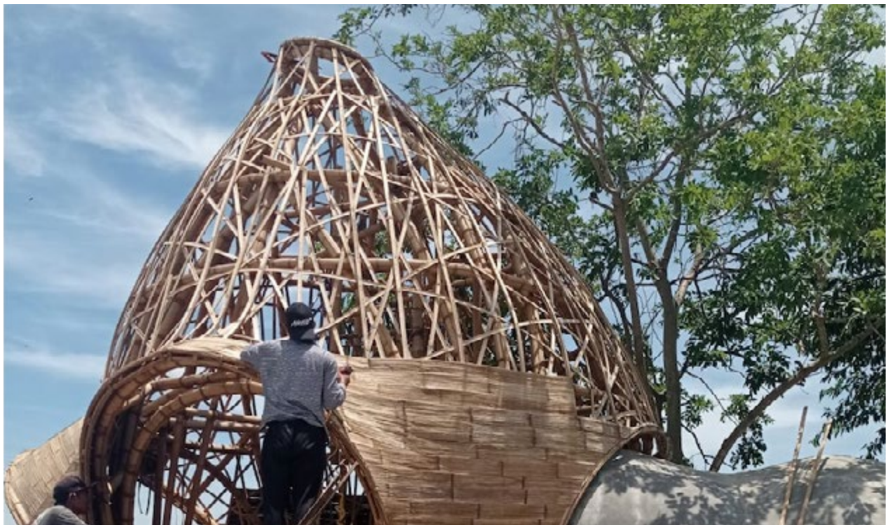
Rafter bamboo splits. K Club ubud - Lobby. Tegallalang, Bali. 2019.
