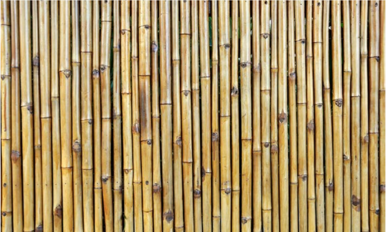
Bamboo Cladding Ø 2-3cm with lasure dove finishing - Bali, 2018.
