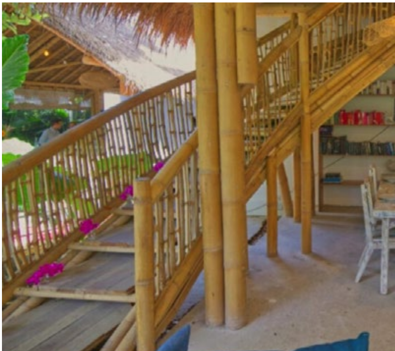
Bamboo stairs & wood steps. Villa Nangka – Gili Air, Bali. 2020.
