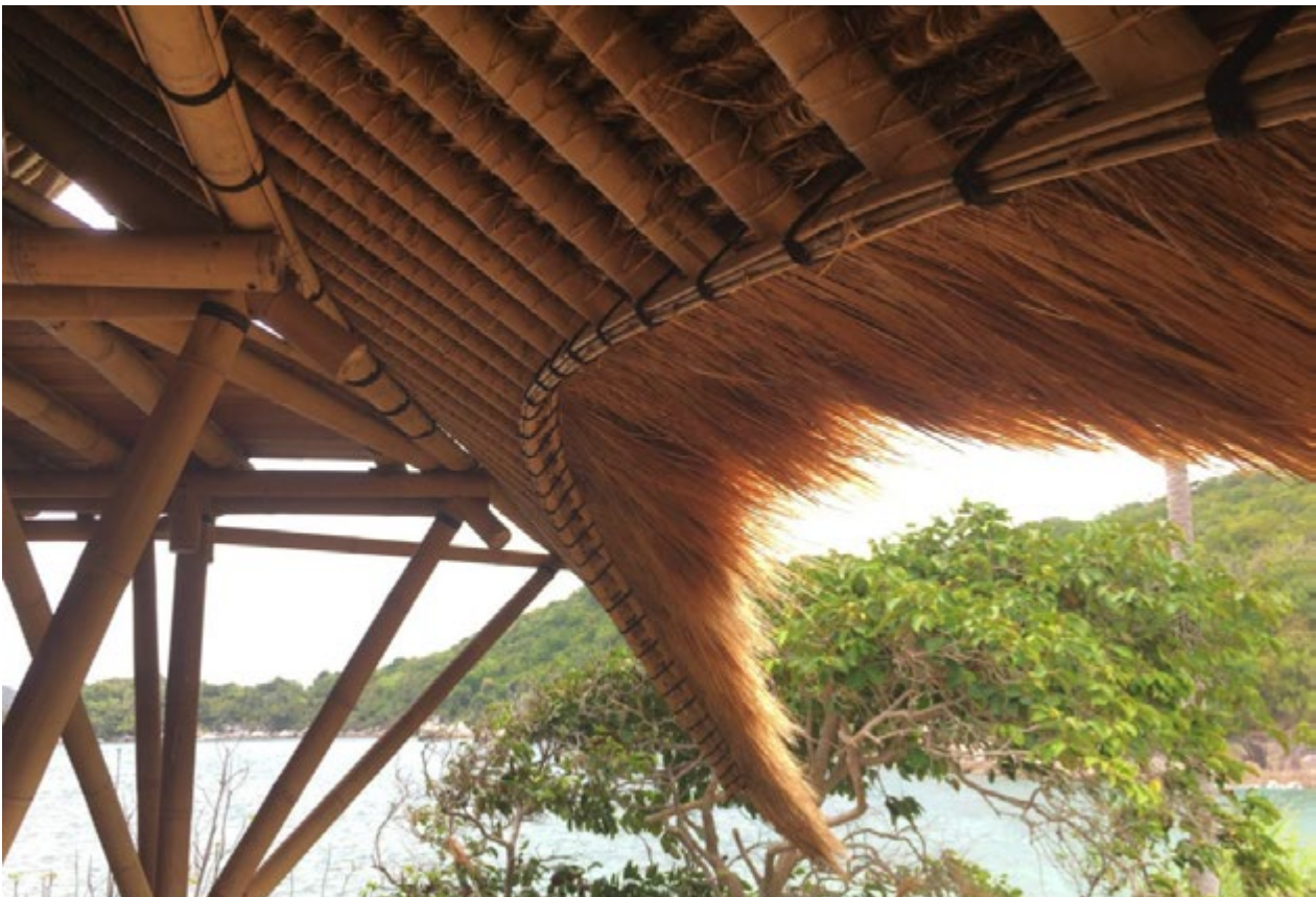
Alang alang roof and split roof edge - Eco Symbiosis, Survival Ecotourism - Anambas, Indonesia. 2018
