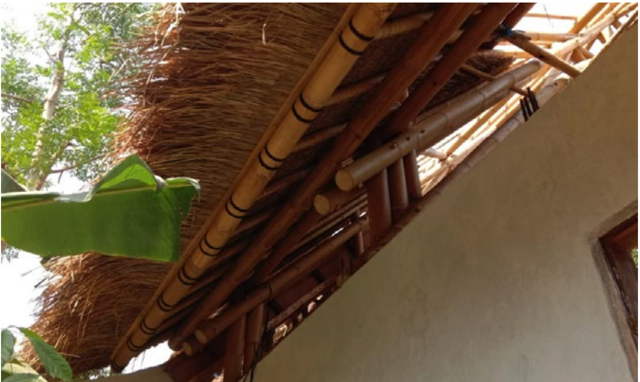
Alang alang roof edge with round bamboo - Villa Nangka, Gili Air, Indonesia. 2019.
