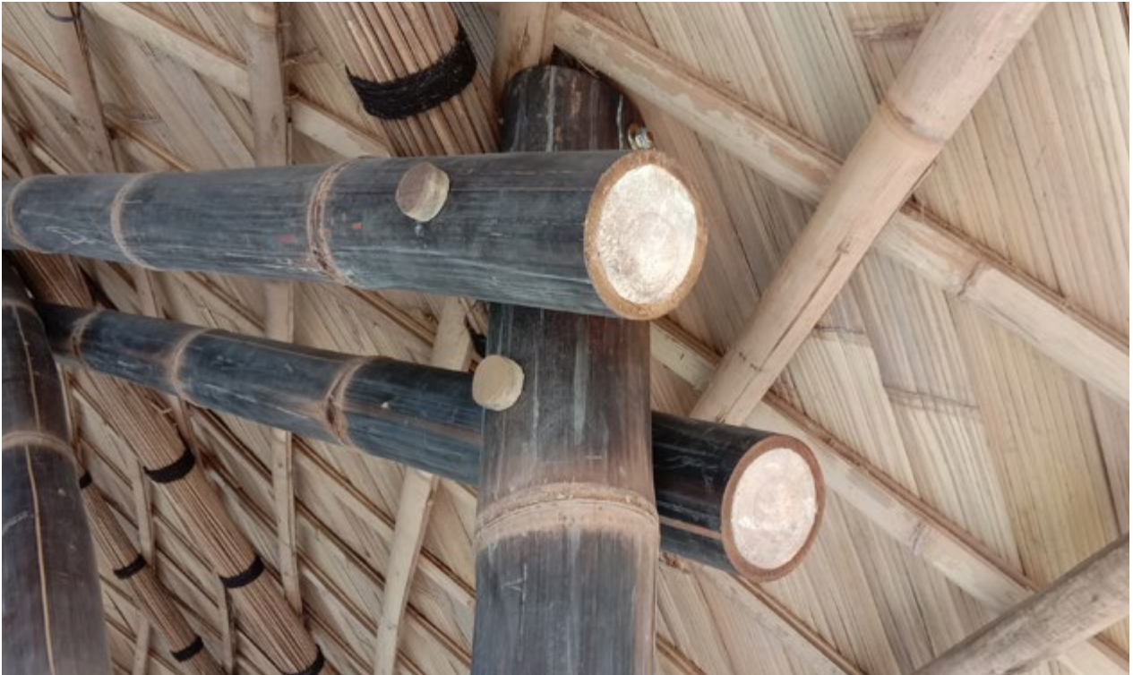
Cover holes with albecia wood (closed and not closed)- K Club – Tegallalang, Bali. 2019.
