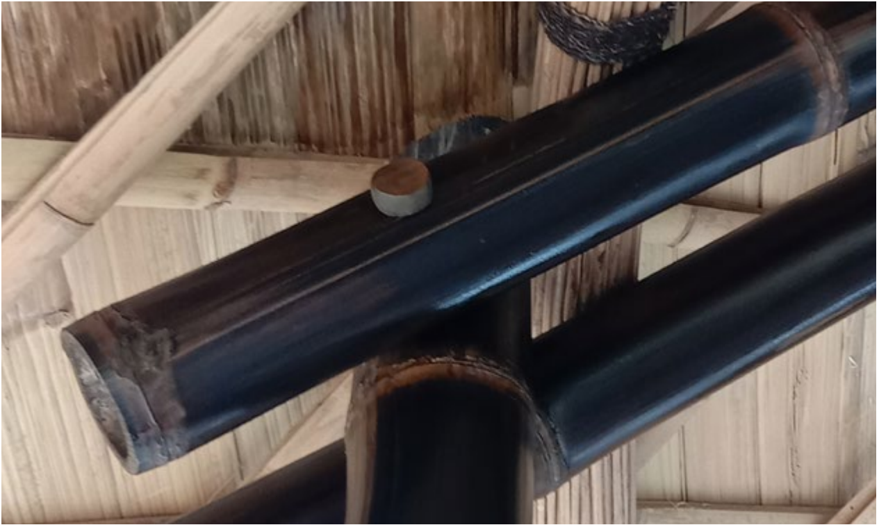
Cover of the steel bars with bamboo petung - Tegallalang - Bamboo Lobby, Bali, 2019.
