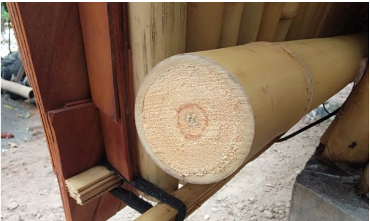
Cover holes with albecia wood before finishing -Restaurant – Candidasa, Bali. 2021.
