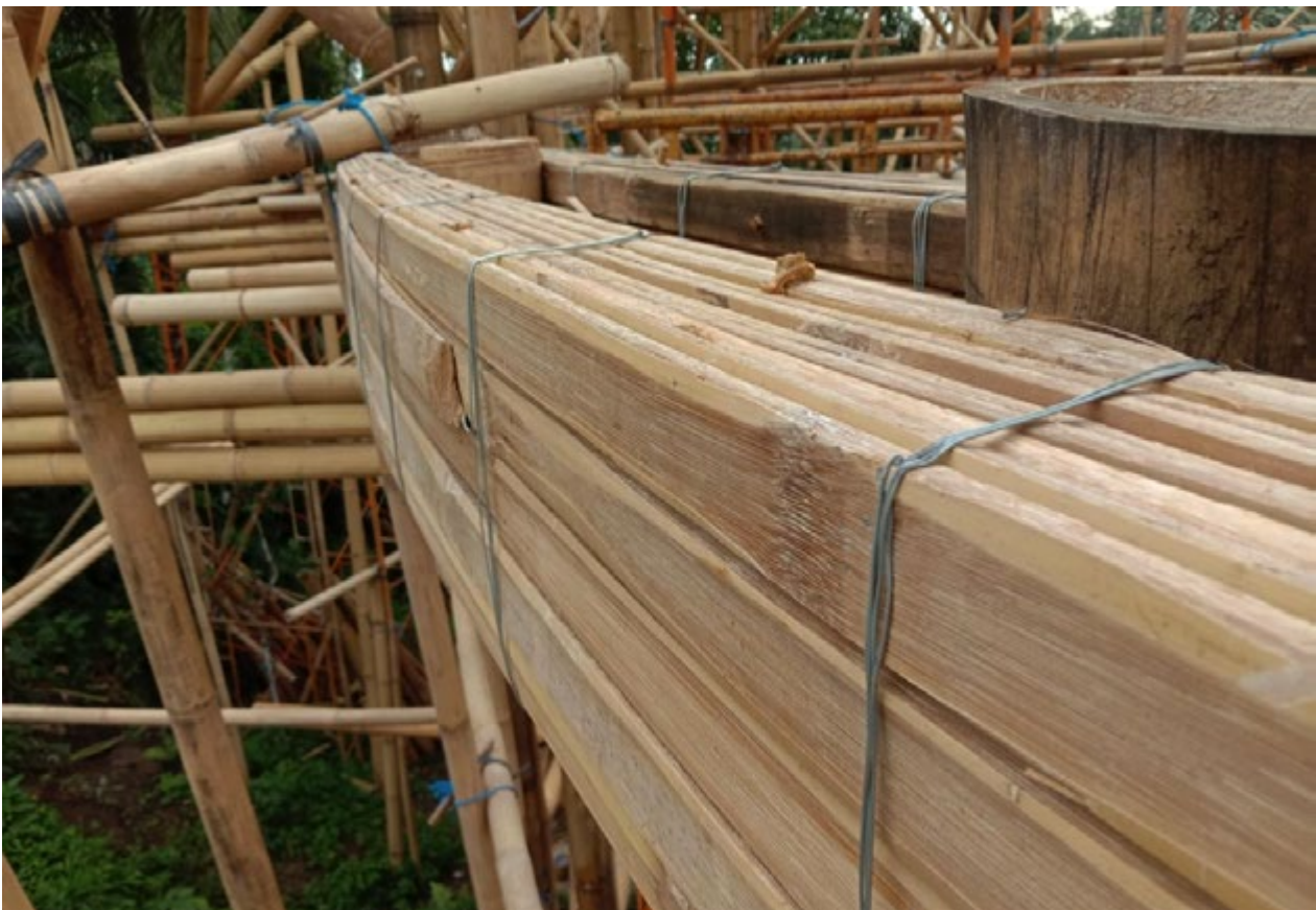
Split beam during construction - Tea House, Ubud, Bali. 2020.
