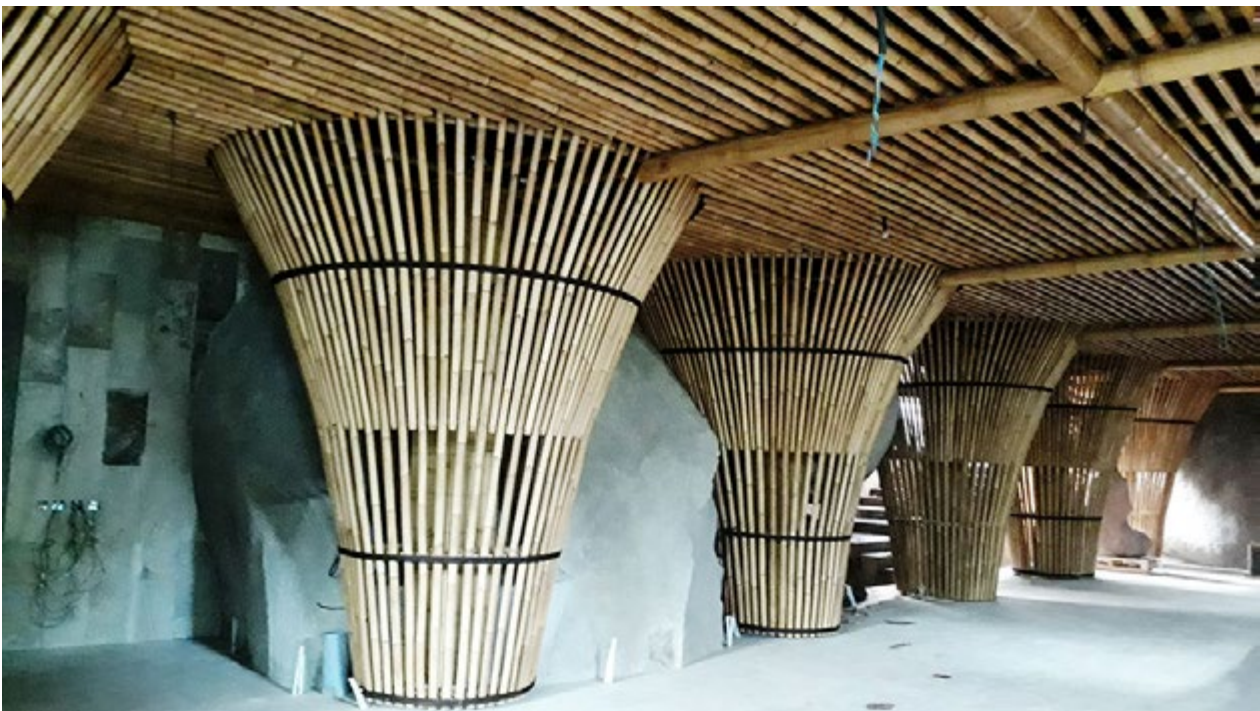
Bamboo tali \varnothing 6-7cm for interior Spa. Kinput, spa – Seychelles Island. 2017.
