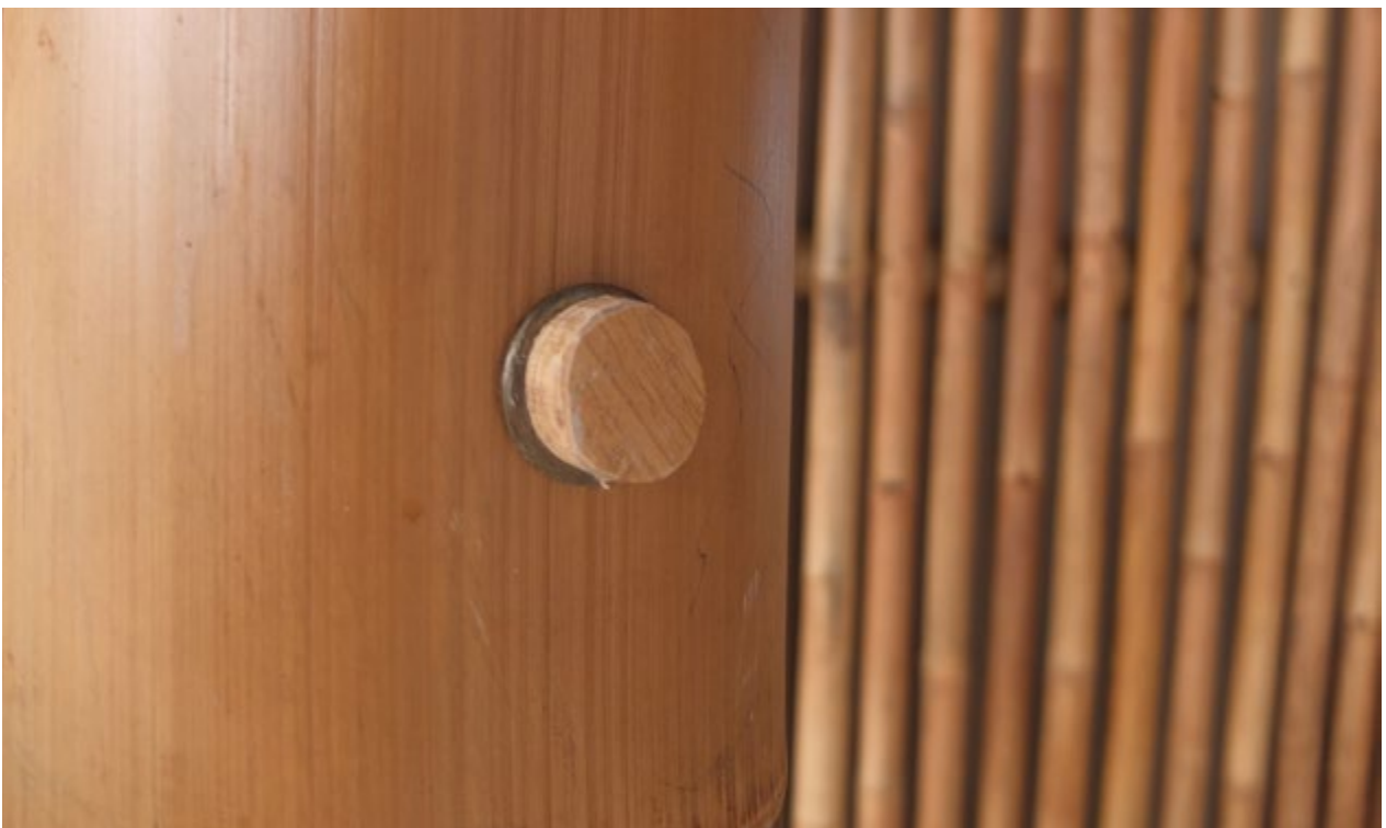
Cover of the steel bars with bamboo caps - Yoga Shala, Joali Being, Bodufushi, Maldives, 2021.
