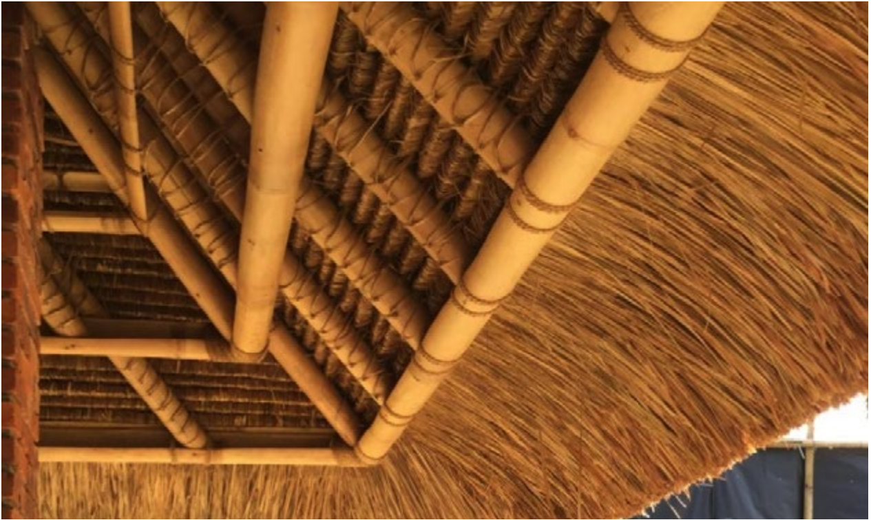
Alang alang roof edge with round bamboo – Mutia Garden Restaurant – Medan, Indonesia. 2019.
