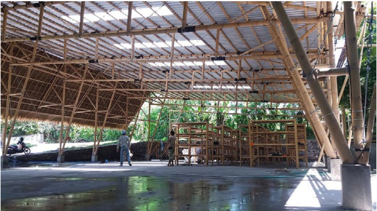
Bamboo petung with concrete pedestal. Warehouse Tripper, Batubulan, Bali. 2015.
