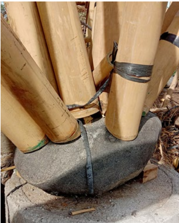
River stone pedestal, Ulaman Eco Retreat, Bali. 2020.
