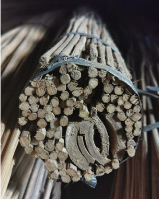
Detail bamboo lidi beam with inside bamboo split to connect with main beams and columns.
